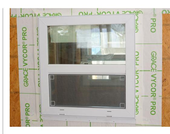
Grace® Vycor® PRO flashing, with its highly conformable film and non-asphaltic, butyl-modified adhesive technology, provides premium protection against water infiltration in all critical non-roof detail areas. Vycor Pro contains no asphalt and is compatible with flexible PVC window flanges and leading sealant technologies.
